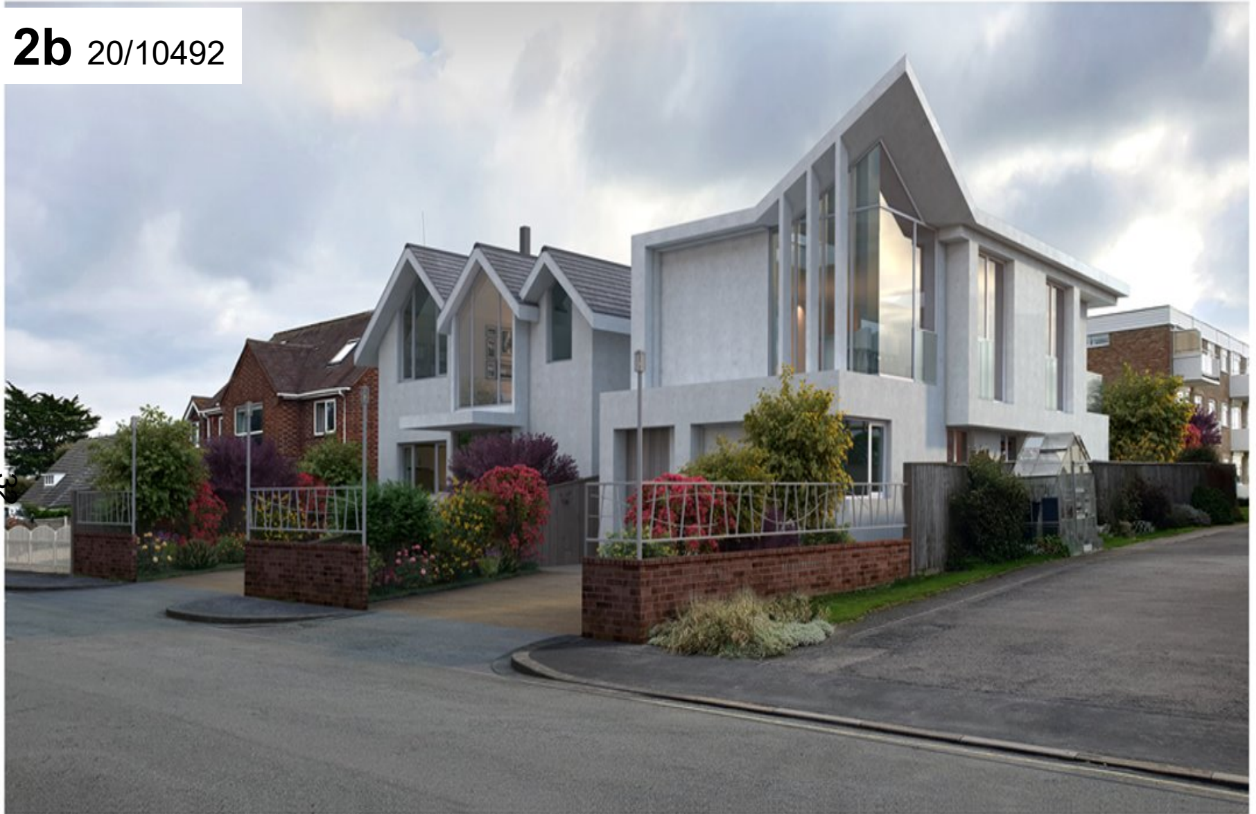
Proposed view from Victoria Road opposite showing the building, landscape, environmental and habitat enhancements. Proposed New House on the Site to the West of Victoria Cottage, Victoria Road, Milford on Sea, SO41 0NL Copyright Visionary Architects Ltd 2019 Drawing NQ Pers-02
